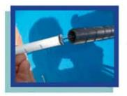
Step 2: Attach Disc & Insert into Riser
